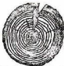
Fig. 58 DRYING CRACK AS SEEN IN CROSS SECTION
