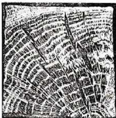
Fig. 56 CROSS SECTION OF A BADLY DRIED OAK-WOOD POST WITH GREAT INTERNAL CHECKS
