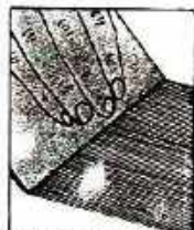
Fig.95. APPLYING GLUE WITH A SPATULAR
